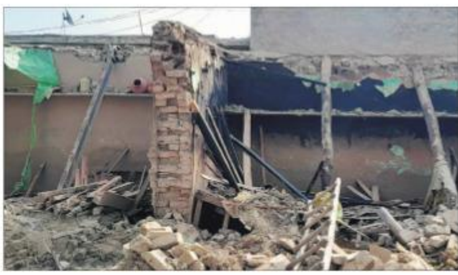
A damaged house in a Ferozepur village. TRIBUNE PHOTO
