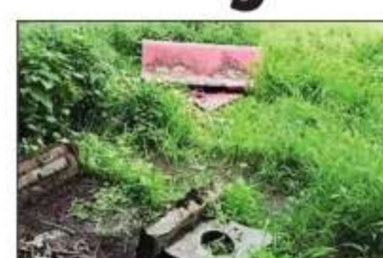
The broken bench at K'ghar park
