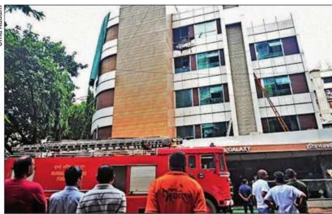
The BMC had recently issued a notice to Hotel Galaxy in Prabh Colony for not adhering to fire safety norms
