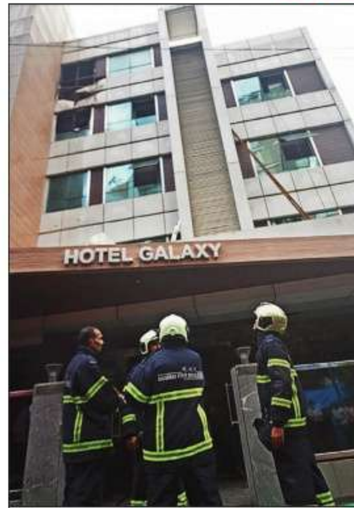
Fire broke out in Hotel Galaxy in Santacruz (E) on Sunday afternoon, killing 3 people
