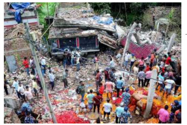
Under ruins: Rescue operations after a blast at a firecracker unit in North 24 Parganas district of West Bengal on Sunday. PTI
